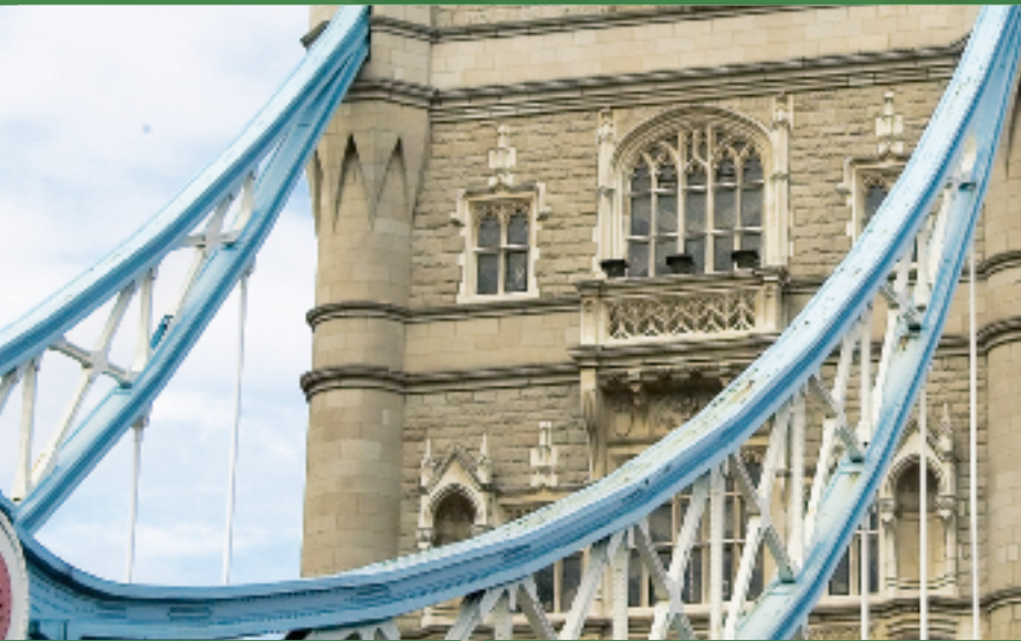
Tower Bridge London, England
